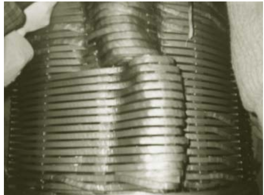
Figure 1 Typical winding deformation found in a scrapped transmission transformer
